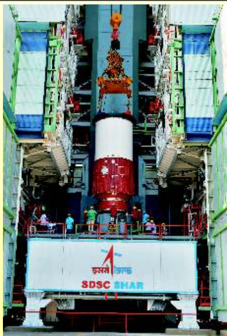
Hoisting of Nozzle End Segment of PSLV-C37 core stage during vehicle integration
