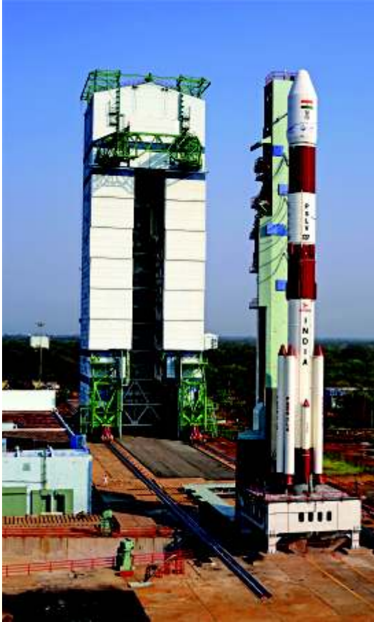
PSLV-C37 at the First Launch Pad
